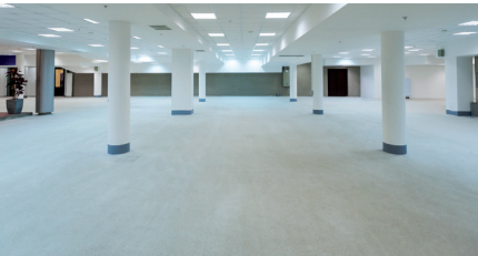
2.1_Thin film system Smooth finish \approx 300 microns thickness
