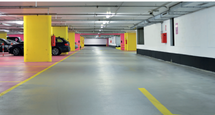
2.2_Thick film system Textured finish \approx 600 microns thickness
