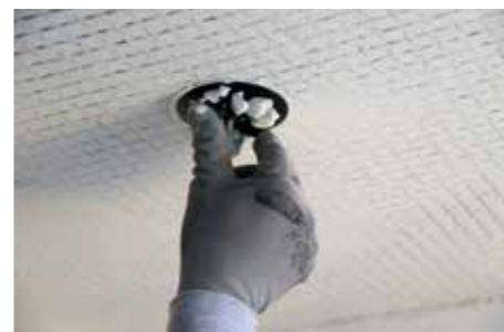
4 Enroscamento de TASSELLO STEEL DRYFIX no varão STEEL DRYFIX.
