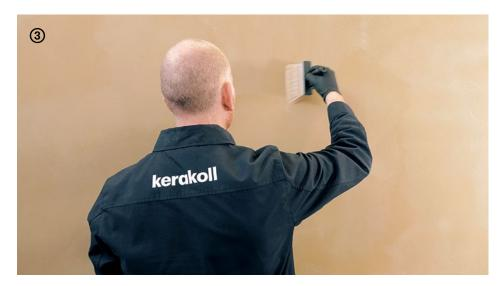
$\rightarrow$  Remove any dust with a dry flat brush or a cotton cloth and then apply the  $2^{nd}$  coat of **Finish**.
