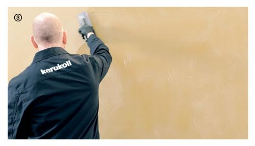
→ Apply the  $2^{nd}$  coat once the material has hardened (3 - 12 hours). Tip: if crests or flashes are present, sand in order to remove them before applying the  $2^{nd}$  coat. A drop of water may be added in order to make the product more workable.
