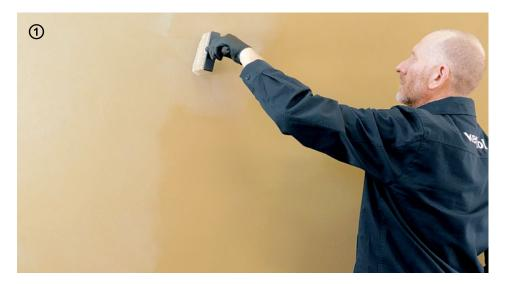
→ Once the coloured texturizing finishing coat Patina has completely dried, apply the 1<sup>st</sup> coat of Finish by brush without sanding.
