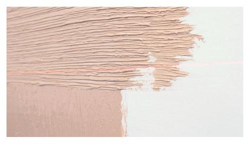
Tip: the use of a laser leveller pointed at the wall might be useful in order to keep the lines perfectly horizontal.
