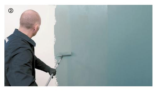
→ Decor must be carefully applied with a roller over the whole surface in 2 coats, either pure or diluted to a maximum of 5 - 10%.
