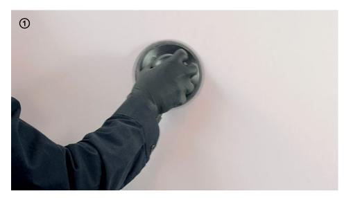
→ Before applying **Decor**, sand the surface with 80-220-grain sandpaper in order to make the surface perfectly smooth and pleasing to the touch.
