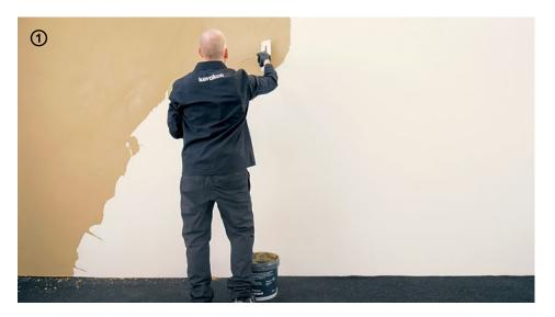
$\rightarrow$  Apply the 1<sup>st</sup> coat of **Patina** spreading the product with small and even strokes of the spreader over the entire surface.
