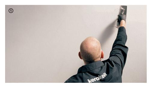
$\rightarrow$  Apply the 1<sup>st</sup> coat of **Wallcrete** spreading the product with small and even strokes of the spreader over the entire surface.
