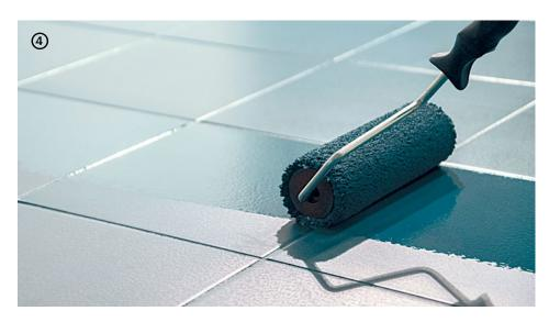
Tip: in overlapping areas, blend together by lifting up the roller, in order not to leave excess amounts of material. When applying in several connected rooms, leave gaps at the thresholds connecting the rooms by using the joints as breaks.
