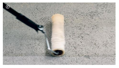
→ The absorbent cement-based substrates must be treated with EP21 applied neat and spread using a roller with a coverage of ≈ 200 ml/m<sup>2</sup>. Tip: flaky substrates must be treated with 2 coats of EP21. The 1<sup>st</sup> coat diluted with Keragrip Eco Pulep up to 30%, the 2<sup>nd</sup> coat, 6 hours later, with pure EP21.
