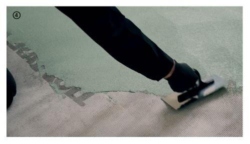
→ Spread the product with a finishing trowel and level to cover the Net 90 mesh, respecting the coverage of ≈ 2.5 kg/m<sup>2</sup>. Pay attention during application to the complete coverage of the glass fibre mesh.
