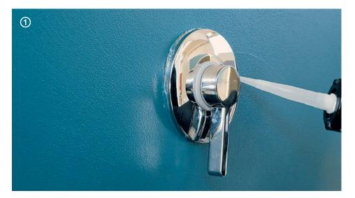
→ After the application, use Hyperflex Hybrid clear transparent sealant or Silicone Color to seal plaques, vents, shower cabinets and drains in environments with frequent contact with water.
