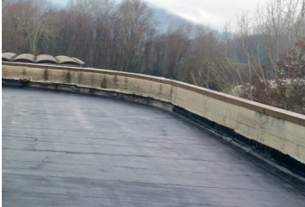
Bituminous rainproof waterproofing system on old sheeting
