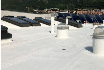
Cool Roof system on old sheeting
