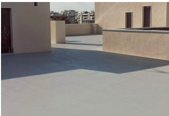
Decorative fibre-reinforced rainproof waterproofing system suitable for foot traffic
