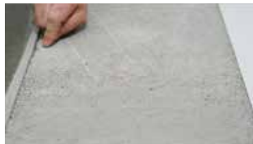
CEMENT-BASED SCREED checking hardness and cleanliness
