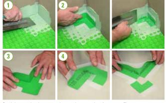
$create\ an\ internal\ corner\ and\ two\ overlapping\ edges.\ Seal\ the\ overlap\ between\ the\ two\ bases\ using\ Aquastop\ Fix.$
