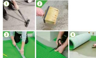
Apply Biogel® gel adhesive using a suitable toothed spreader; lay a thin layer with the smooth side, pressing down heavily to achieve maximum adhesion to the substrate and regulate water absorption.
